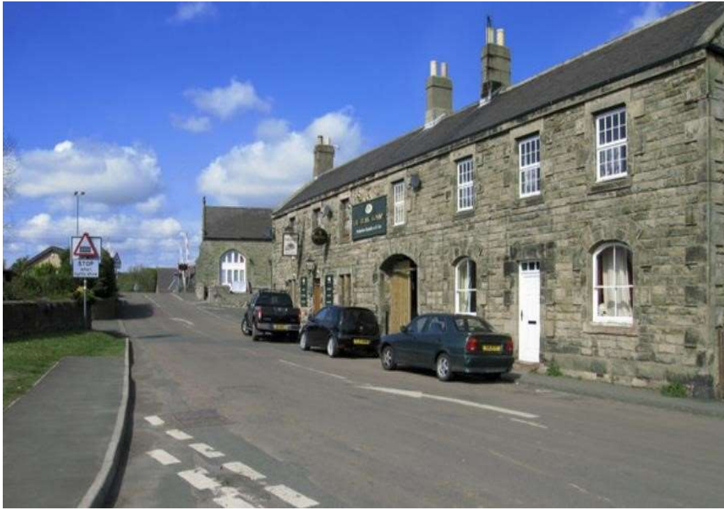
Figure 2: Typical building styles in Christon Bank
